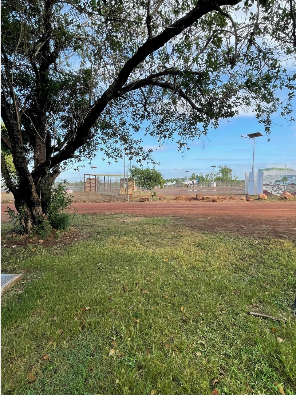
Figure 4: Tamarind Park showing the road crossing with existing toilet block in the background. Approximate sewer trench location path.
