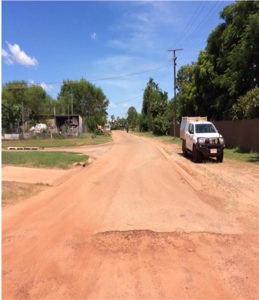
Intersection at Sayle Court
