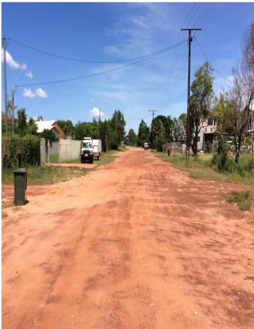
No kerbing or gutter
