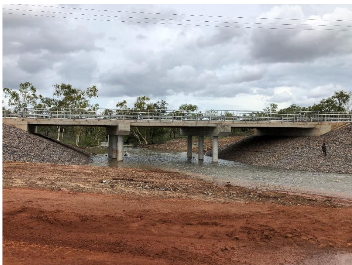
Rocky Creek Bridge in the final stages of construction.
